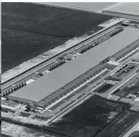
Google Data Center Netherlands
